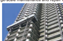
Lift Climber Mast-climbing work platform for large-scale maintenance and repair work
