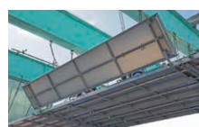
SPIDER PANEL Panel-type hanging scaffolding system
